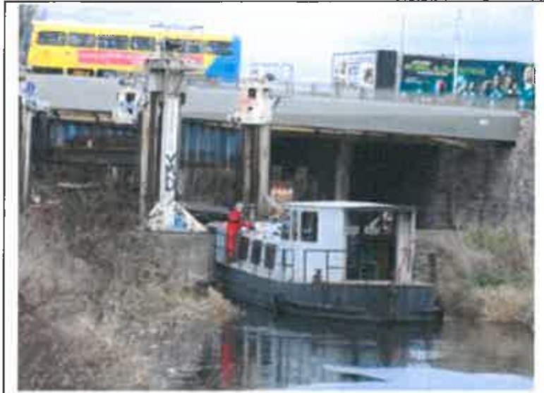
Caption: The 'Effin' Bridge, above Spencer Dock, Dublin. Barge 118B beginning its passage under the rail bridge, elevated on four jacks by Irish Rail staff, just below Lock 1 on the Royal Canal.
