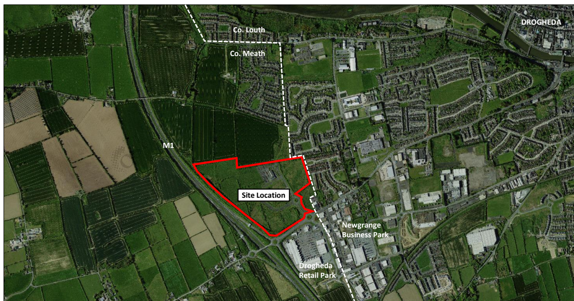
Figure 1: IDA Business and Technology Park, Donore Road, Drogheda
